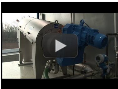
Video: HUBER Screw Press Q-PRESS@ - here at a municipal WWTP https://www.youtube.com/watch?v=5VsPNKbkJyA
