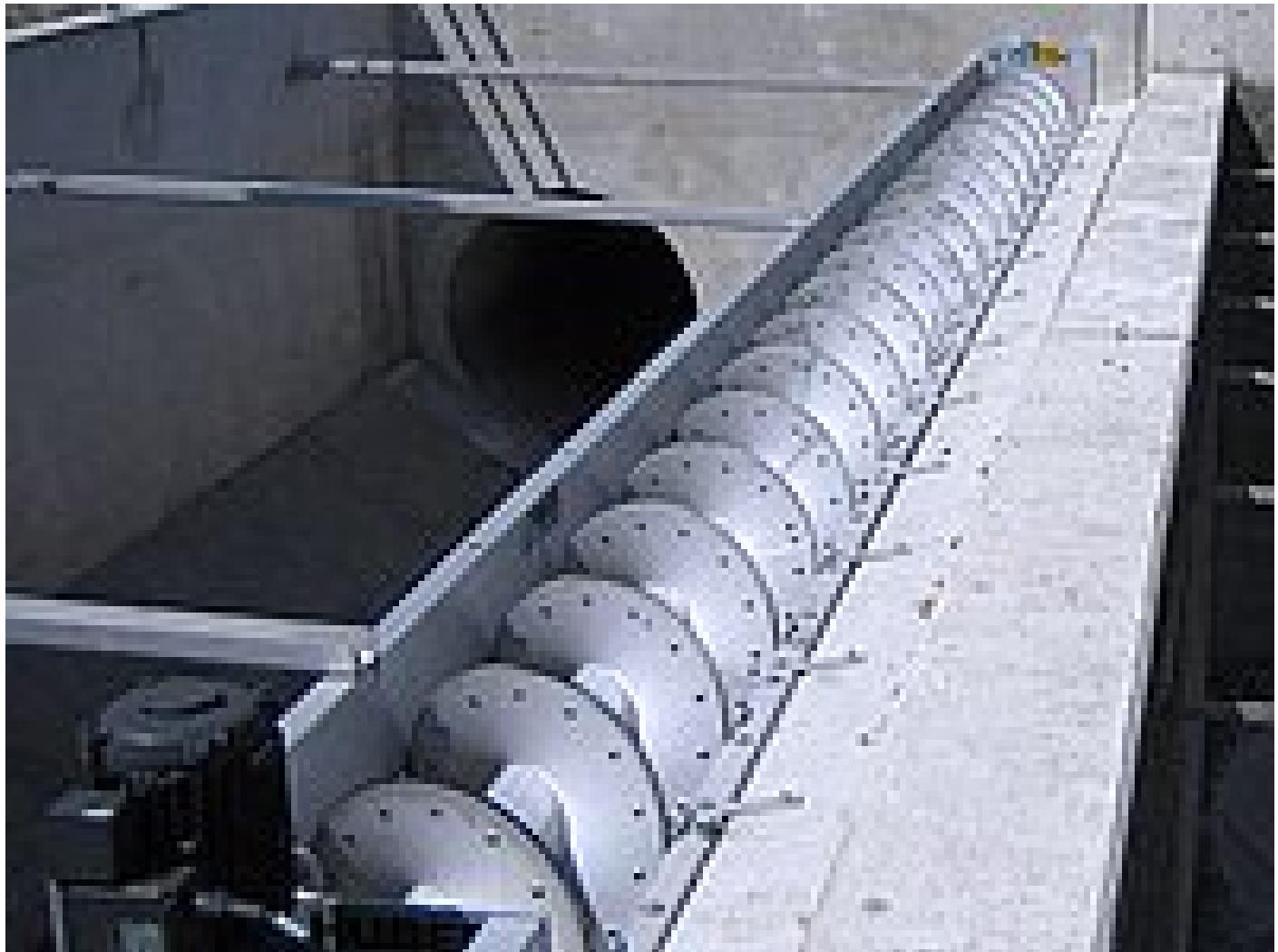
Automatically cleaned screen for solids retention in stormwater tanks and overflows
