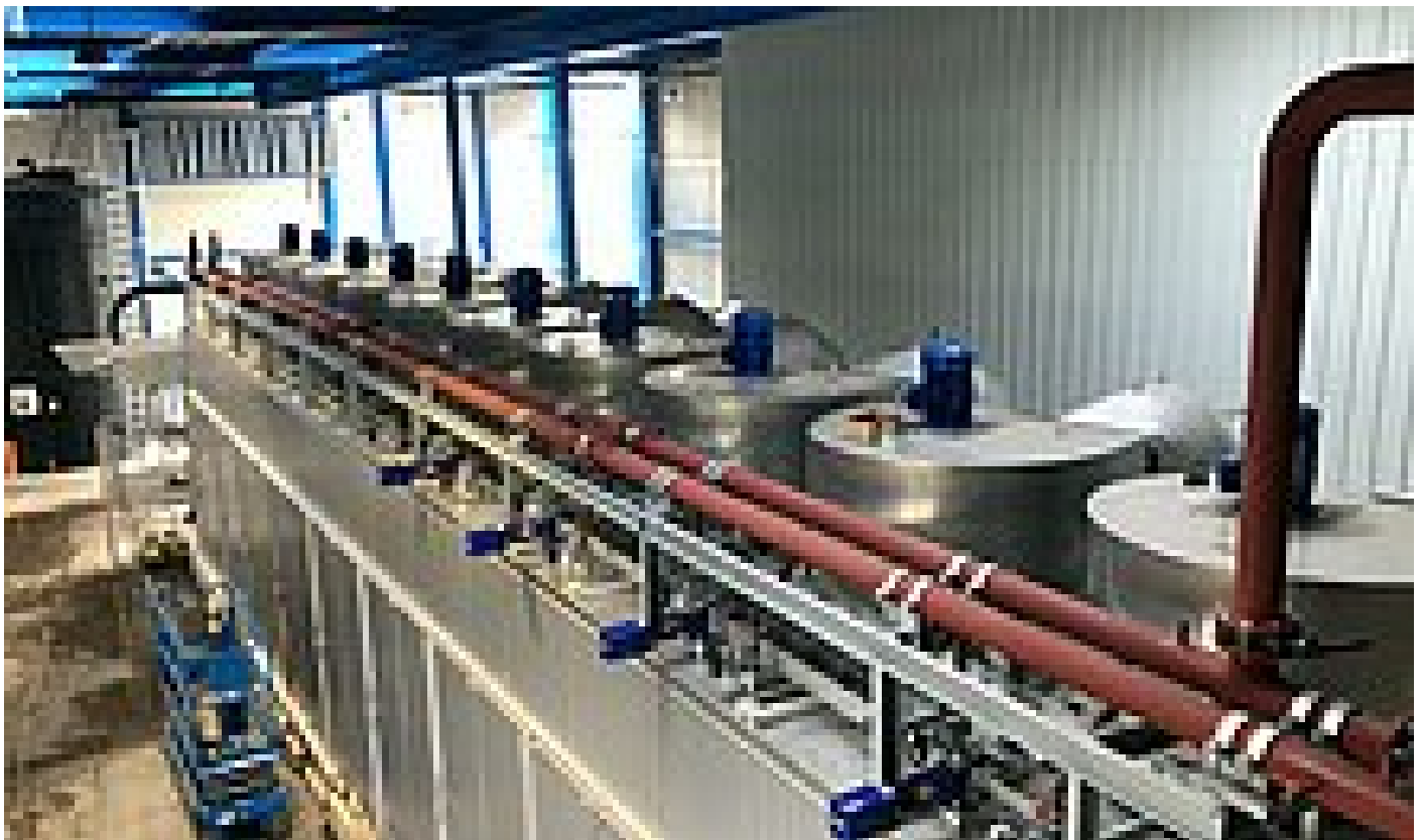
Assembly of the HUBER BT 20 belt dryer
