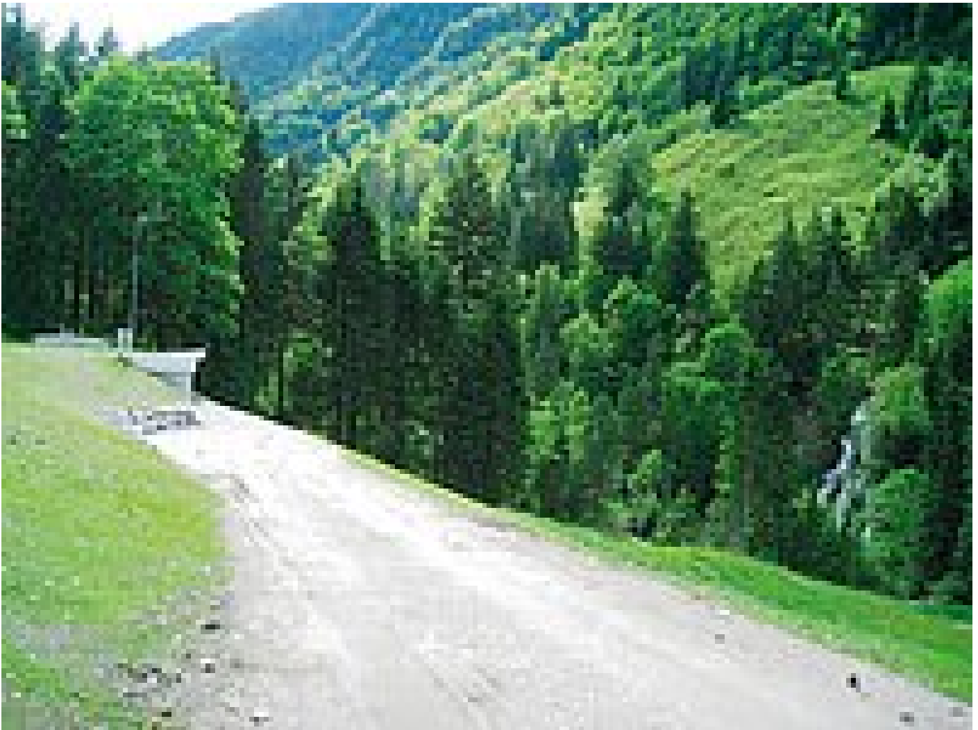
The inlet structure on the left, the spring overflow on the right
