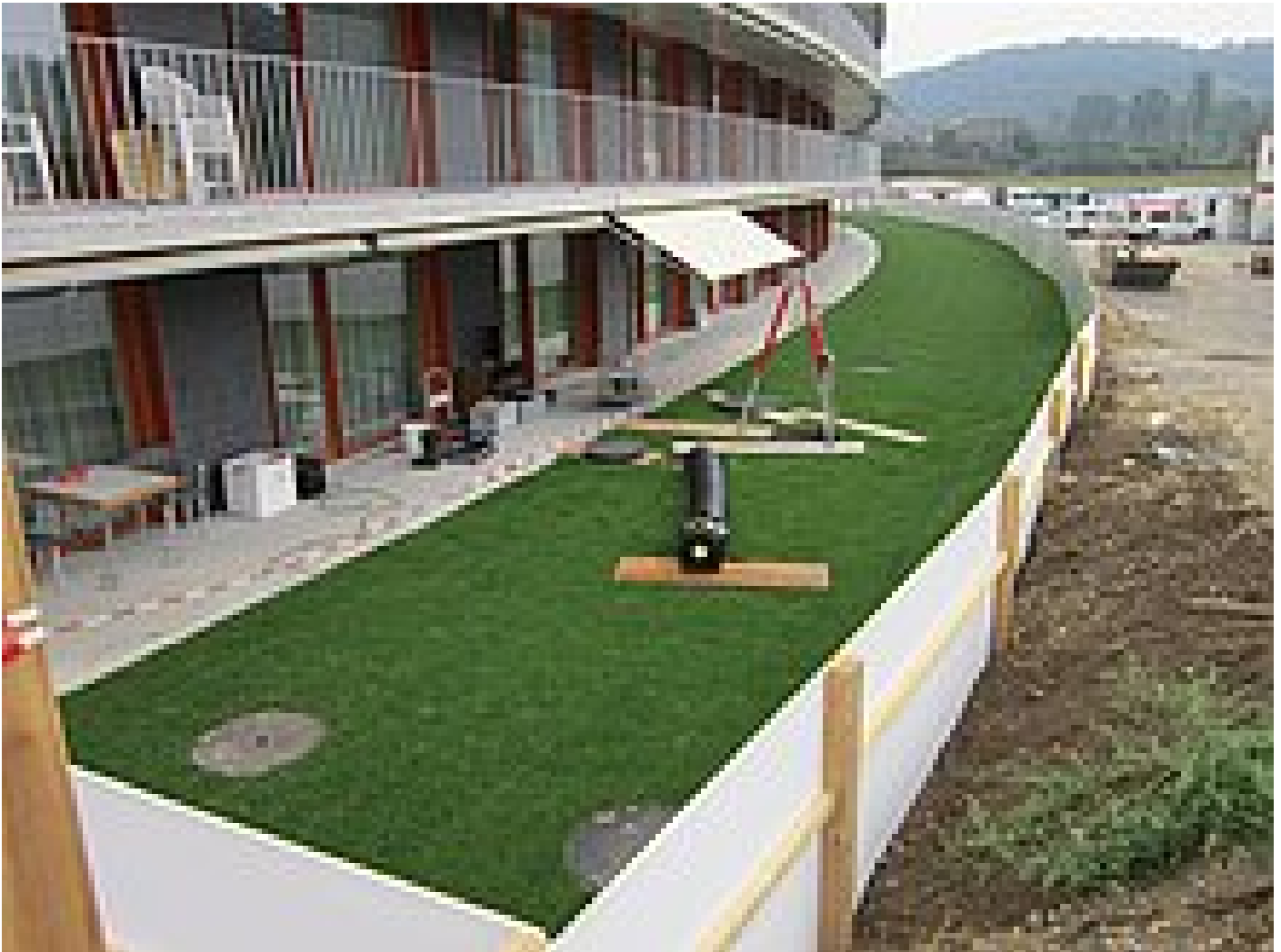
Figure 1: Old-age home Hofmatt in Münchenstein after the first stage of modernisation with the entrance to the wastewater shaft in the garden
