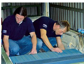
Repairs carried out by our experienced service staff on site or in the HUBER Service factory repair shop
