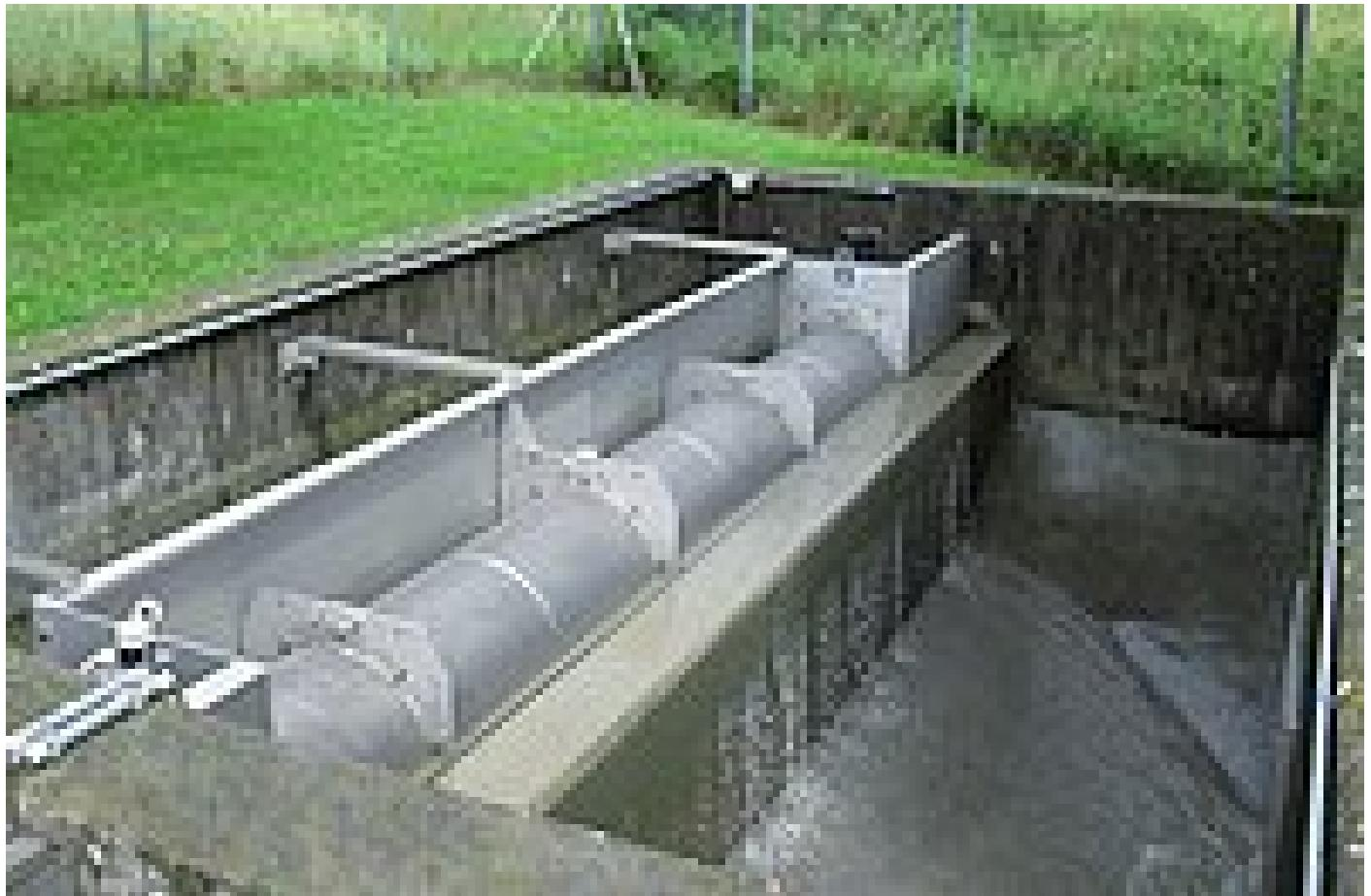
Automatically cleaned screen for solids retention in stormwater tanks and overflows
