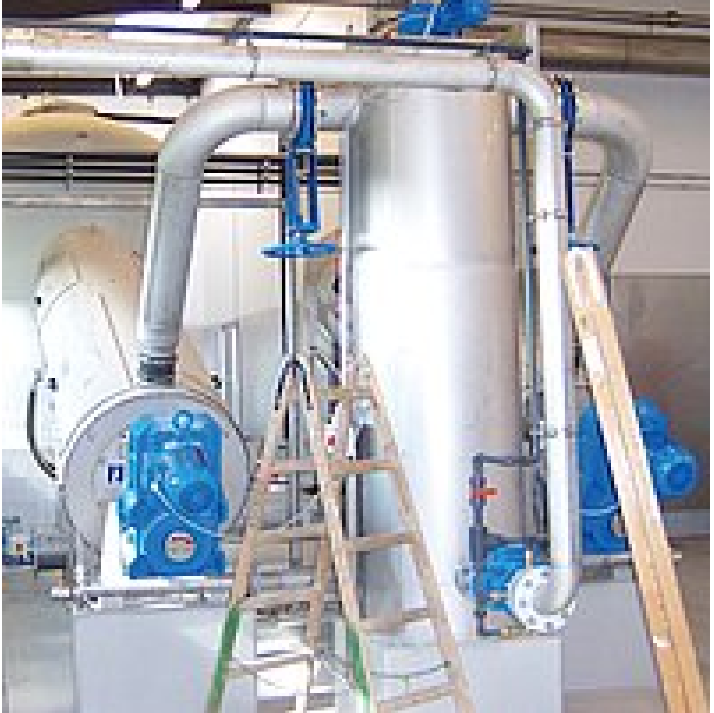
ROTAMAT® flotat sludge dewatering RoS3/3 with flocculation reactor
