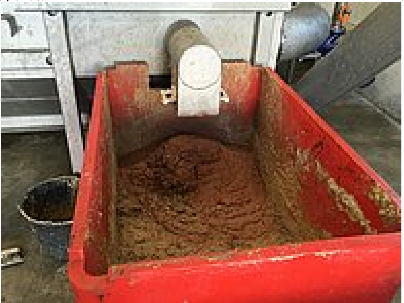
Discharge from the fat separation
