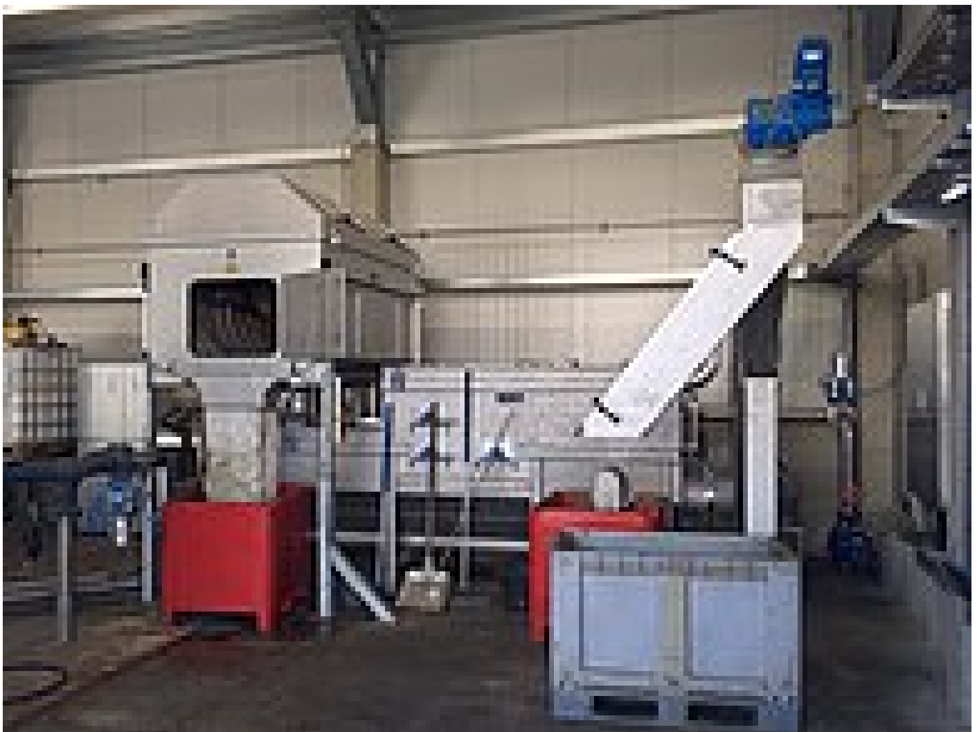
HUBER Drum Screen RoMesh® 3 and HUBER Longitudinal Grit Trap ROTAMAT® Ro6 30 with integrated grease paddle
