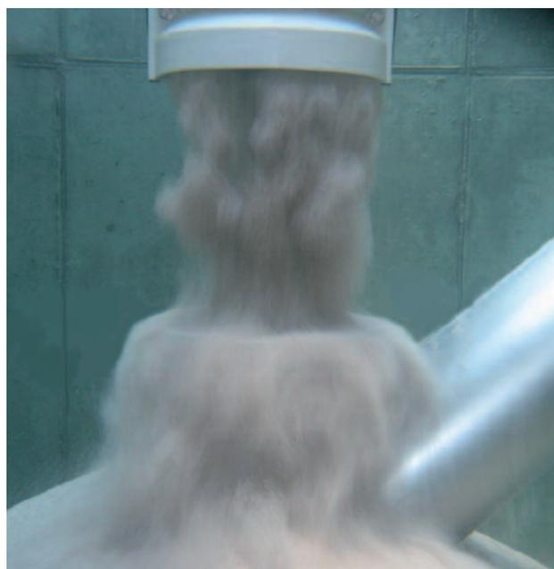
*Crystal-clear effluent from the sandfilter*
