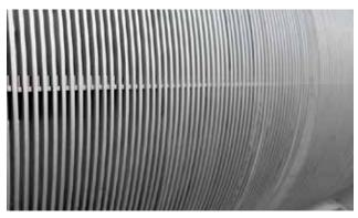
The rake tines, fully engaging with the bar rack, prevent jamming of solids in the bar spacings.
