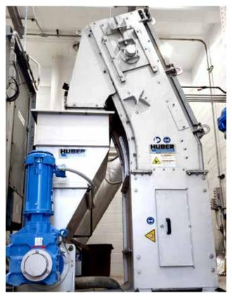
The RakeMax<sup>®</sup> CF combines the benefits of maximum free screen surface and very high separation efficiency. Moreover, it is space-saving and reduces civil costs.
