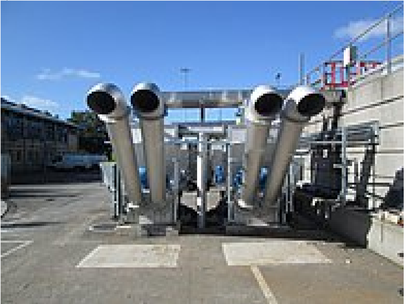
4 off WAP-SL-12 units with a throughput capacity of 15 m 3 /h raw screenings each for highest dewatering efficiency, with a quality factor for screenings < 20 mg BOD 5 /g DR
